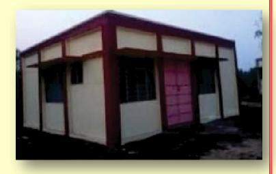
Fig. 2 : A model 2 BHK bamboo reinforced concrete house constructed in school premise near IIT in 2014
