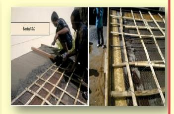
Construction at IPIRTI, Bangalore with Bamboo reinforcement
